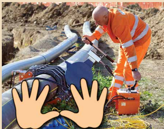
Manual Welding Cycle
